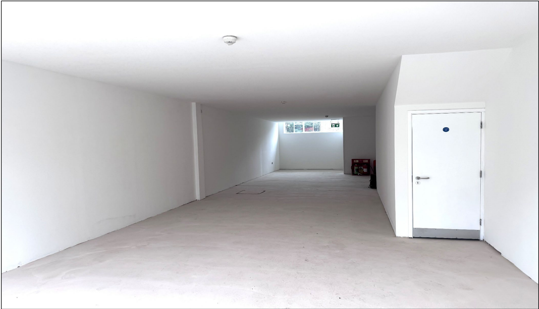
Ground Floor Retail Area
